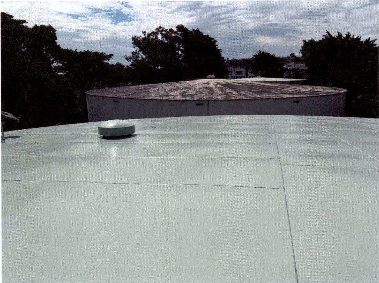
July 1, 2026 – Exterior roof additional top coat.
