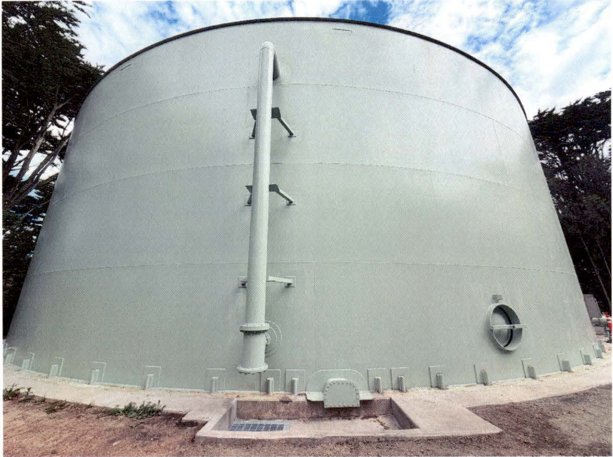
July 17, 2026 – Final tank site post construction – south view.
