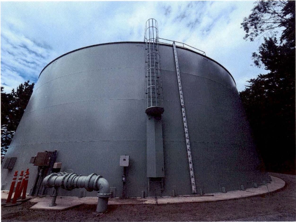
July 17, 2026 – Final tank site post construction – east view.
